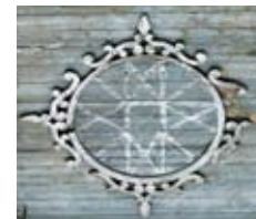
Fragment of the façade of the church
