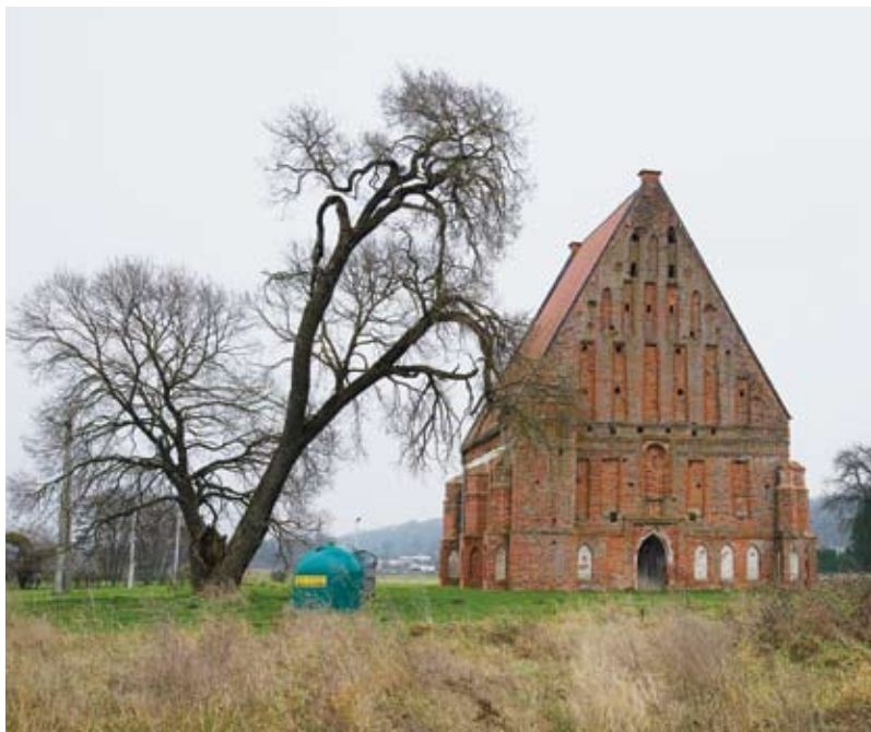
The façade of the old Zapyškis Church
